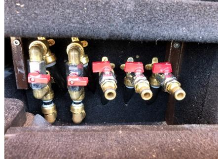
To draw water from a jerry can for showering close the tank 1 & 2 Valves and connect the jerry can hose to the fill valve. After use shut fill valve and open tank 1 & 2 to flush out any remaining shower water.
